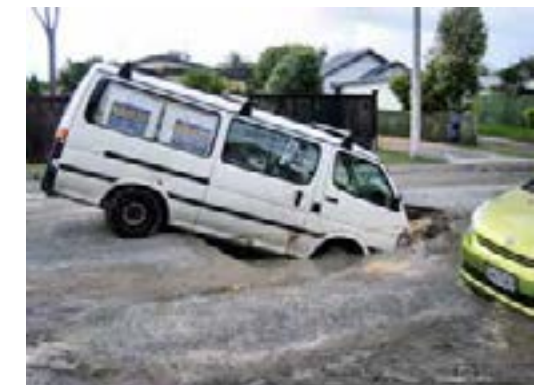
Figure 3.21 Soil liquefaction after an earthquake in New Zealand.
